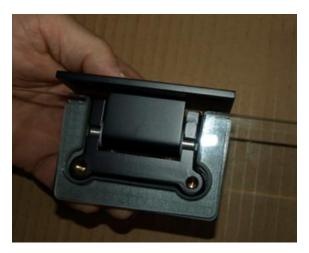
7. Remove the hinge plate and two of the four gaskets (one slightly thicker and one thinner) and position the hinge in one of the cut outs of the glass, so that the two bolts will eventually face in the direction you prefer. Most people prefer to have the screws facing into the bathtub so that the flush side of the hinge is what is seen from the bathroom.
