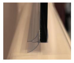
It is important to install the shower screen with a gap between the bottom of the glass and the tub ledge, wide enough to enable the seal to function properly. The design gap is a little over 3/8" (10mm) and it is recommended that the gap be no less than 3/8".
