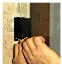
16. Once the shower screen is secured to the wall, ease the shims/spacers out from underneath the glass.
